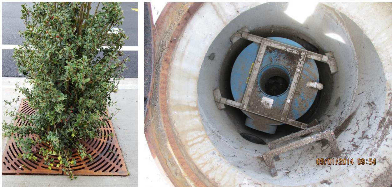
Figure 4.11. Filterterra Units (left) and Filter Cartridge Units (right) are examples of proprietary Treatment devices that meet the requirements of this Design Manual.
