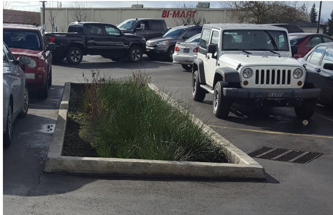
Figure 3.2 Stormwater Planter.
