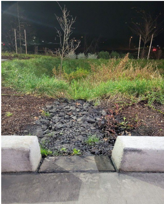
Figure 4.1. An established Rain Garden on a commercial lot, view from an inlet (left), and looking into the facility inlet (right).
