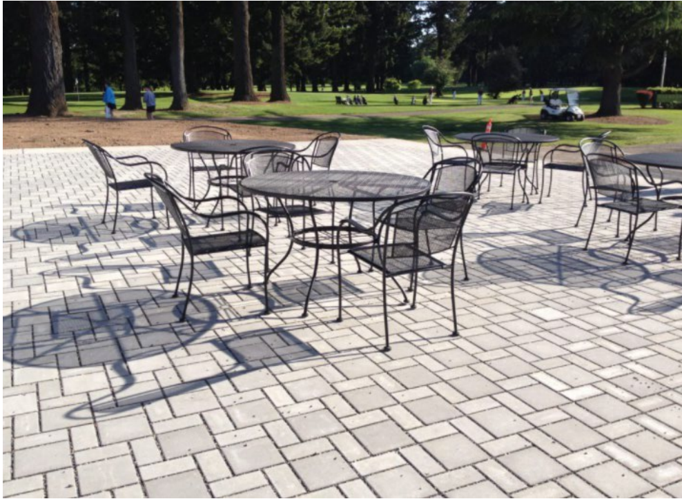
Figure 3.3. Pervious surface not intended for vehicular use.
