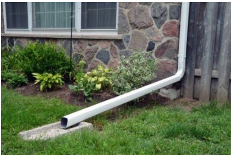
Figure 4.9. Disconnected Downspout to a Pervious Surface
