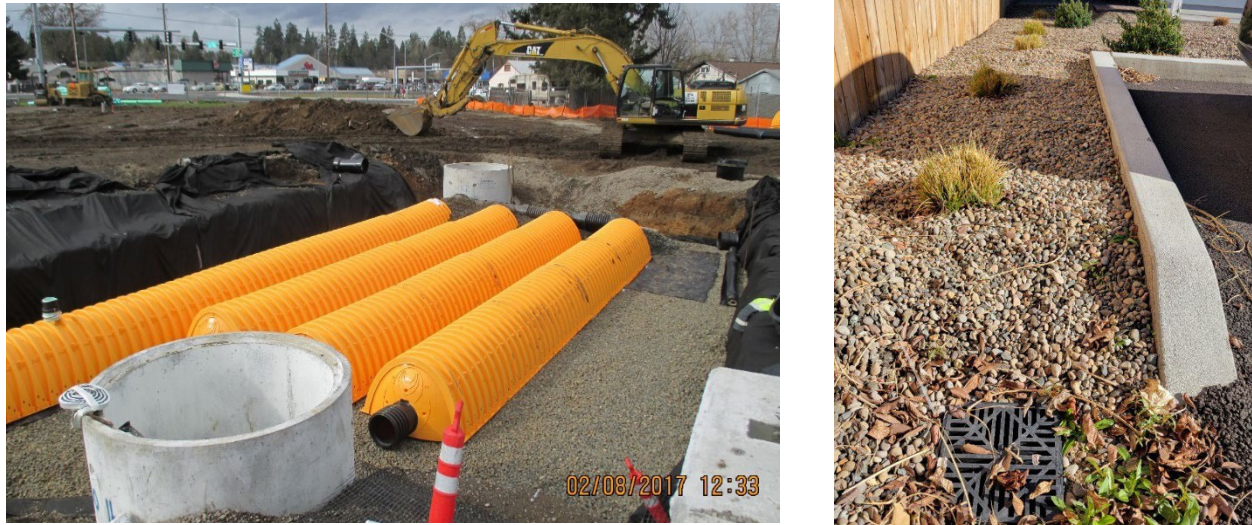
Figure 4.4. Underground chambers (left) are one example of underground Retention when designed to fully infiltrate the Retention storm. Underground Retention can also be designed under a landscape area (right).
