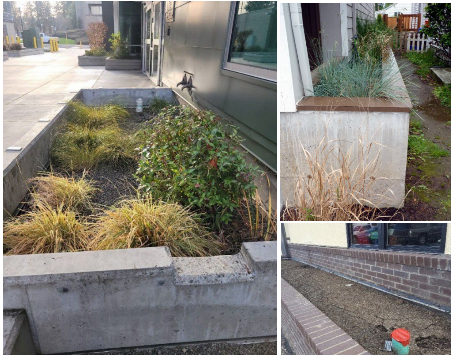
Figure 4.5. Stormwater Planters located flush with a public building (left), a fully-lined residential above-ground Stormwater Planter with an underdrain (upper right), and a newly constructed above-ground Stormwater Planter with an underdrain (lower right).
