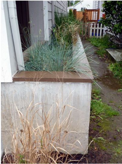
Figure 4.7. A residential above-ground stormwater planter (left). An in-ground stormwater planter with concrete check dams in a public street before planting (right). The centerline (looking straight up the center of this photo) slopes at less than 1%. Concrete check dams were needed because the street slopes more than 1%. Grades parallel to the check dam are flat.
